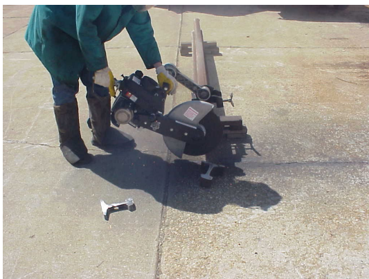
Finishing Rail Cut
