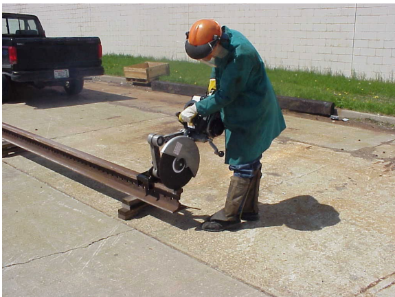
Rail Top Cutting Method
