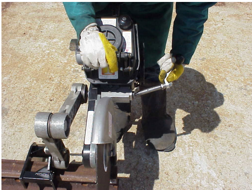
Saw Crank Installing
