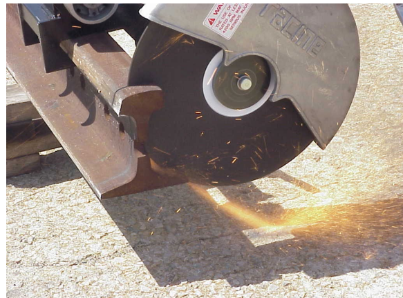
Rail Side Cutting Method
